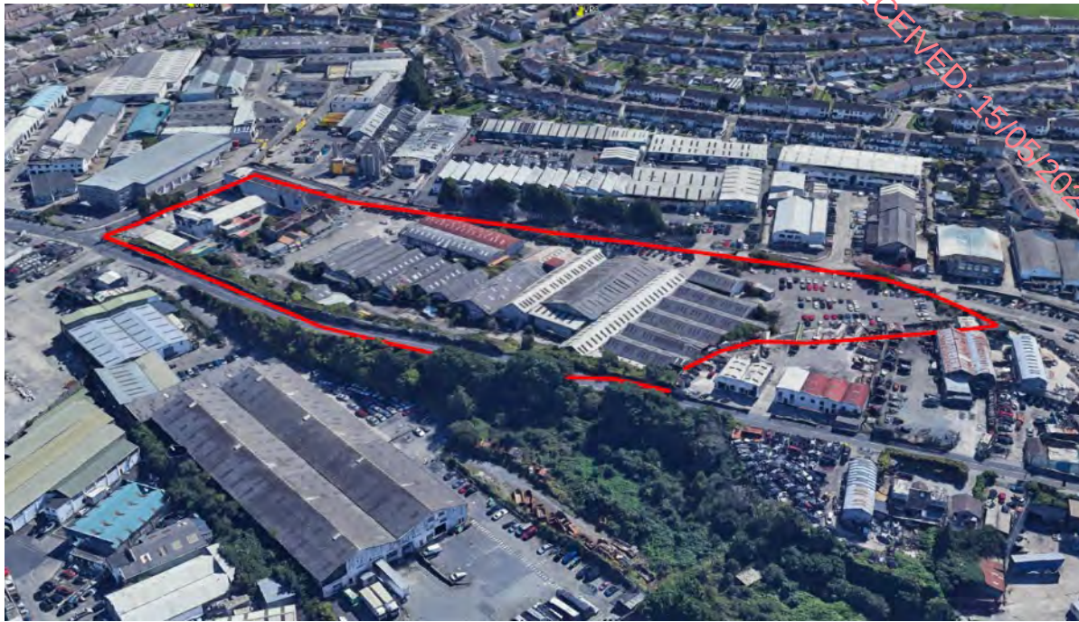
Photo 16.7 Aerial View of Application Site demonstrating existing land-use and townscape setting
